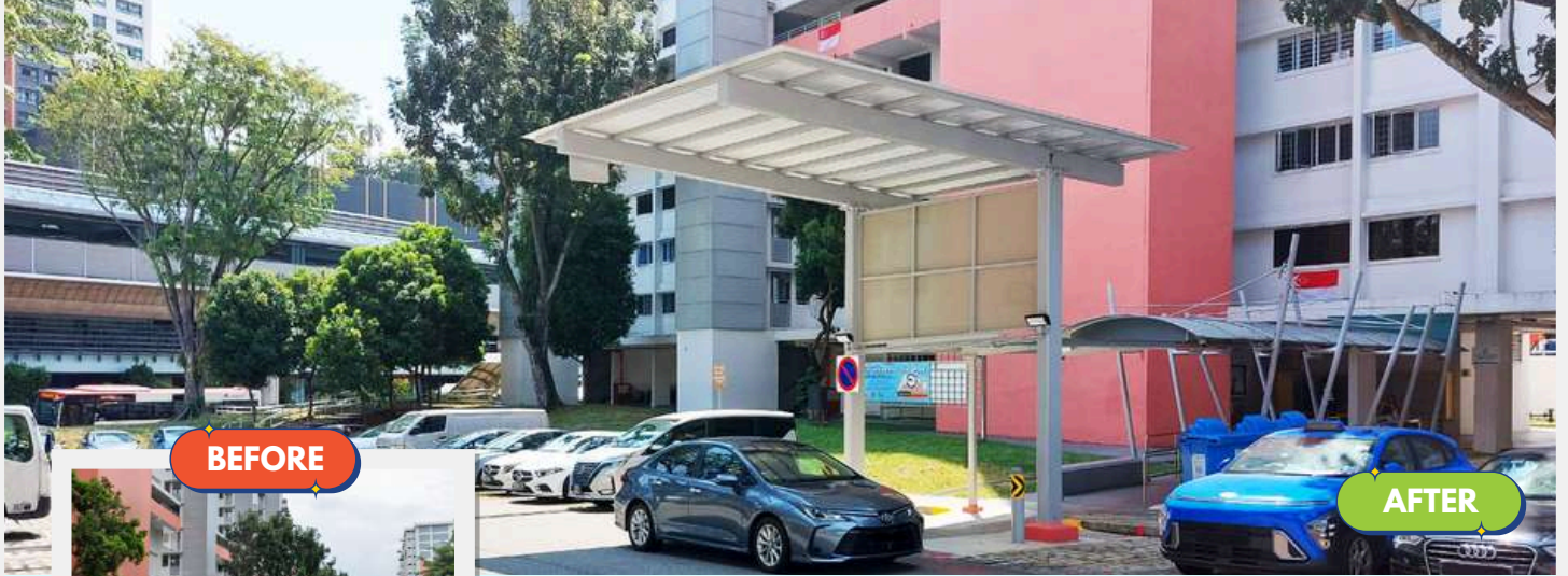
Upgraded Drop-Off Point at Blk 324 Clementi Ave 5
