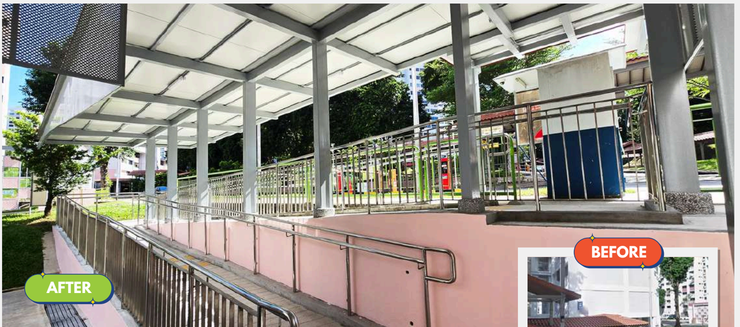
New Sheltered BFA Ramp at Blk 350 Clementi Ave 2
